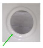
Use plumber's putty or silicone to seal the top of the basin
