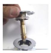
Refit the new plunger and dome and screw into the waste body.
